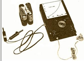
A stand alone receiver having a similar appearance to the Merkur powered by two in series connected  $4\frac{1}{2}V$  batteries. It was mentioned as used with the Sirius III transmitter.
